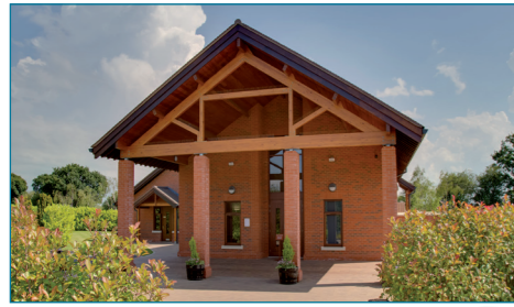
Vale Royal Crematorium, Northwich
